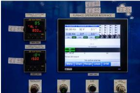
Touchscreen controls and graphic-userinterface simplify operation and remove the need for manual intervention by an operator. Recipes are pre-programmed by the engineering team, and the process is fully automated.
